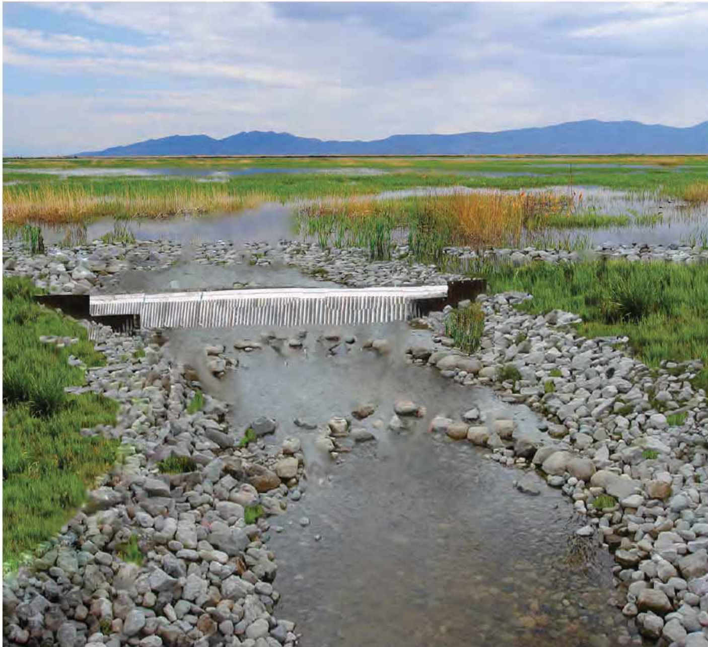
Figure 19. Artists rendering of a typical outflow channel with a picket fish-passage barrier installed. This configuration, or something similar could be used to limit movement of invasive predatory fish like pike or musky.
