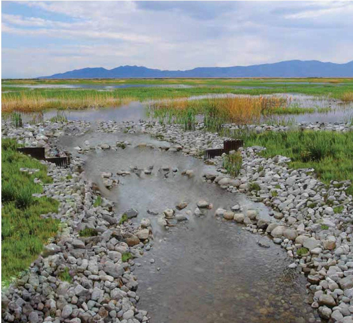
Figure 18. Artist's rendering of a typical outflow channel, looking upstream toward the delta. The loosely-organized arching rock structures will help to slow velocities and promote fish passage when lake levels are lower than the lowered dike.
