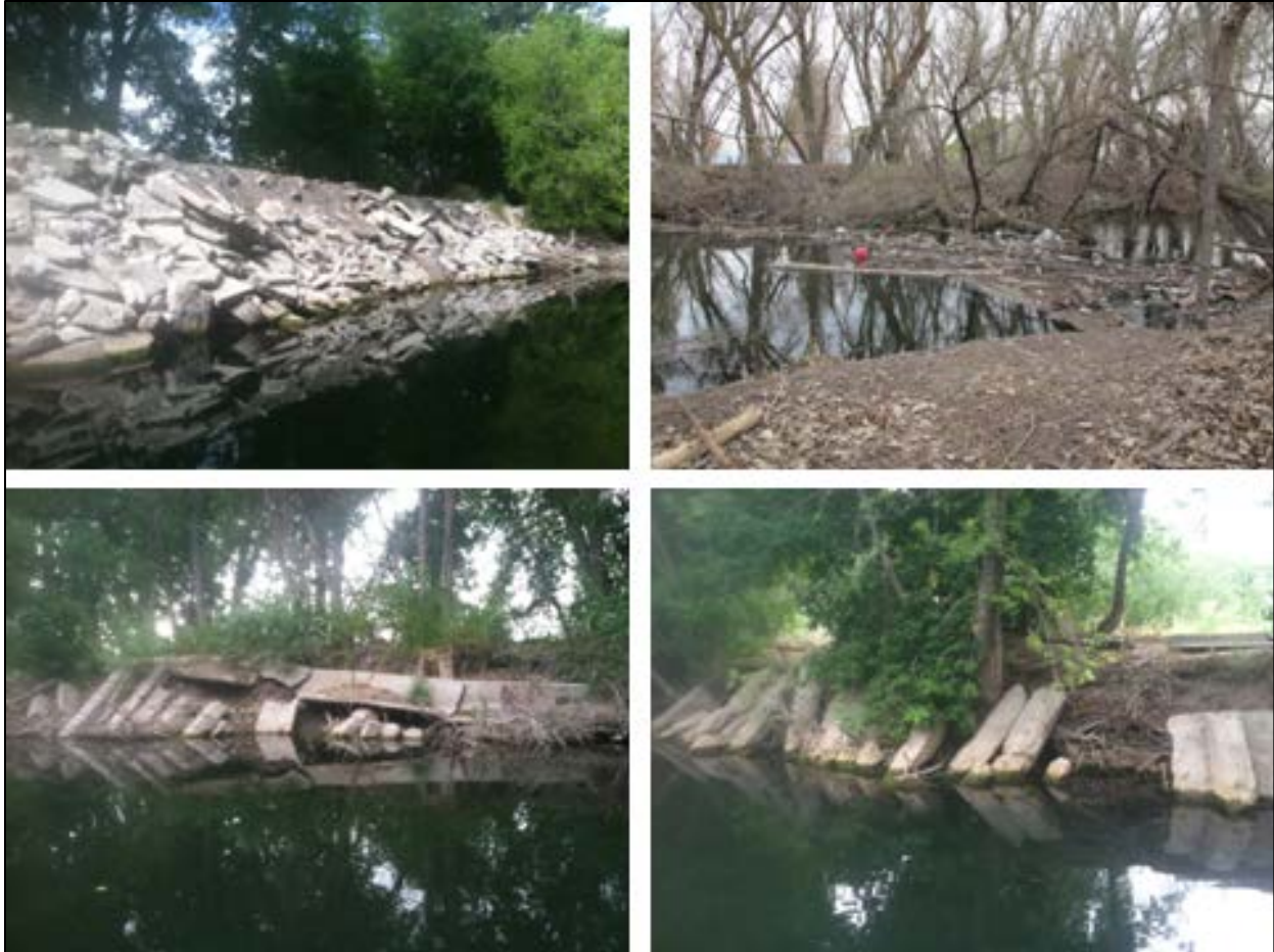
Figure 3-27. Steep banks covered in concrete and trash accumulations are common along the existing river channel. The top left photo shows the existing steep concrete covered south bank just downstream of the Utah Division of Wildlife Resources fish weir. The top right photo shows trash and organic debris accumulations in the existing channel. The bottom photos show the trail and steep concrete covered northern bank downstream of Alligator Park.
